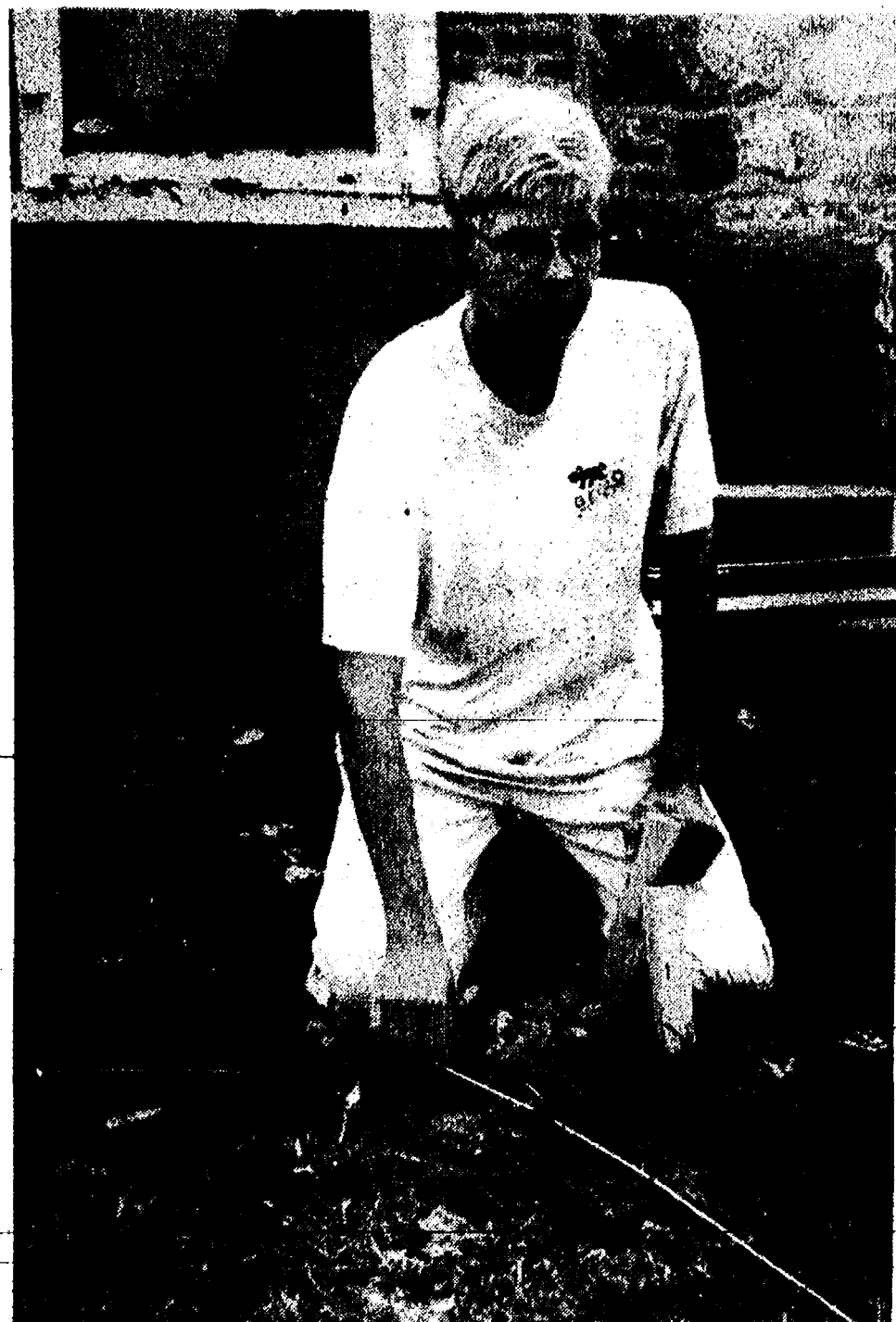
KARSTEN LIPIEC lines up a string to determine how far from the Waterloo Farm Museum farmhouse fill dirt should be applied. Lipiec organized the project for the museum as one of the final stages for becoming an Eagle Scout. The fill dirt will help water drain away from the building, which should alleviate moisture problems the house has had in recent years. Lipiec, who figures to become an Eagle later this year, has to write a paper about the project. Applying the fill dirt was only one portion of the over-all project.
